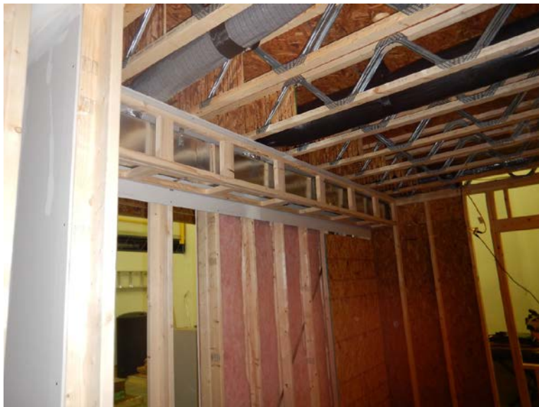
Figure 23. Trunk duct in chase
