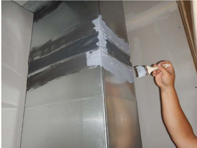
Figure 20. Plenum sealing
