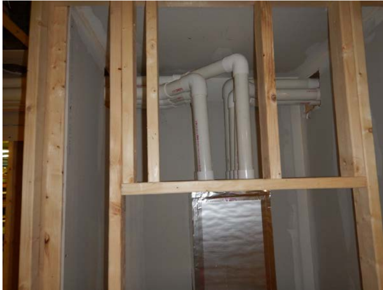
Figure 27. Final connections at plenum manifold
