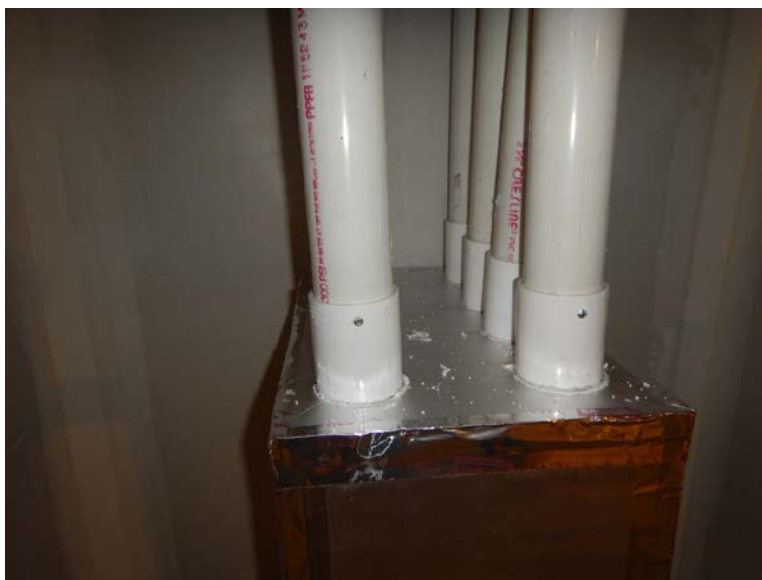
Figure 24. Plenum manifold with takeoffs
