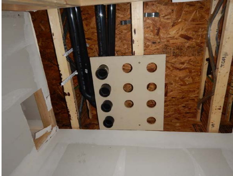
Figure 30. Ceiling support guide
