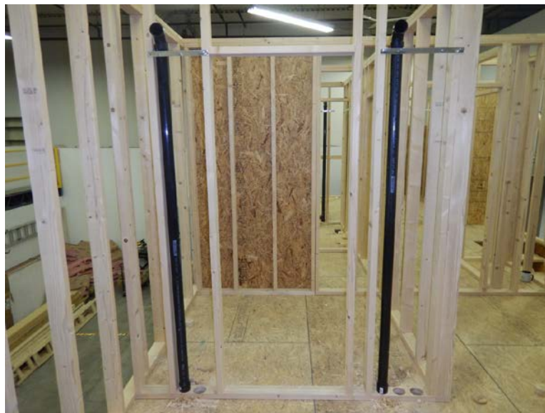
Figure 29. High-sidewall outlets
