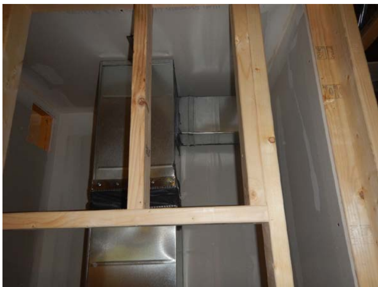
Figure 18. Riser plenum and side takeoff
