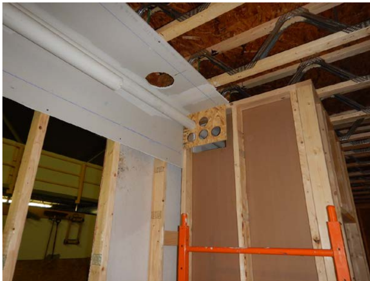
Figure 26. Pipe support blocks
